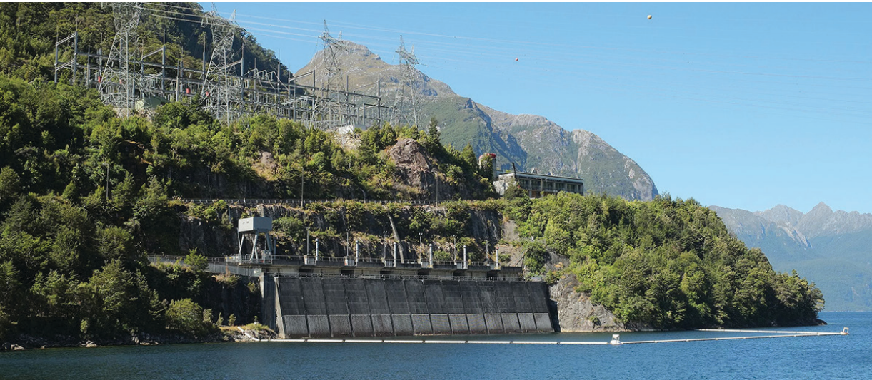
Manapouri power station at Lake Manapouri Image Pseudopanax
