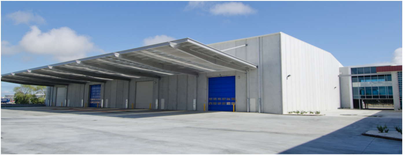
Figure 11. Rocklabs' new facility from the outside
